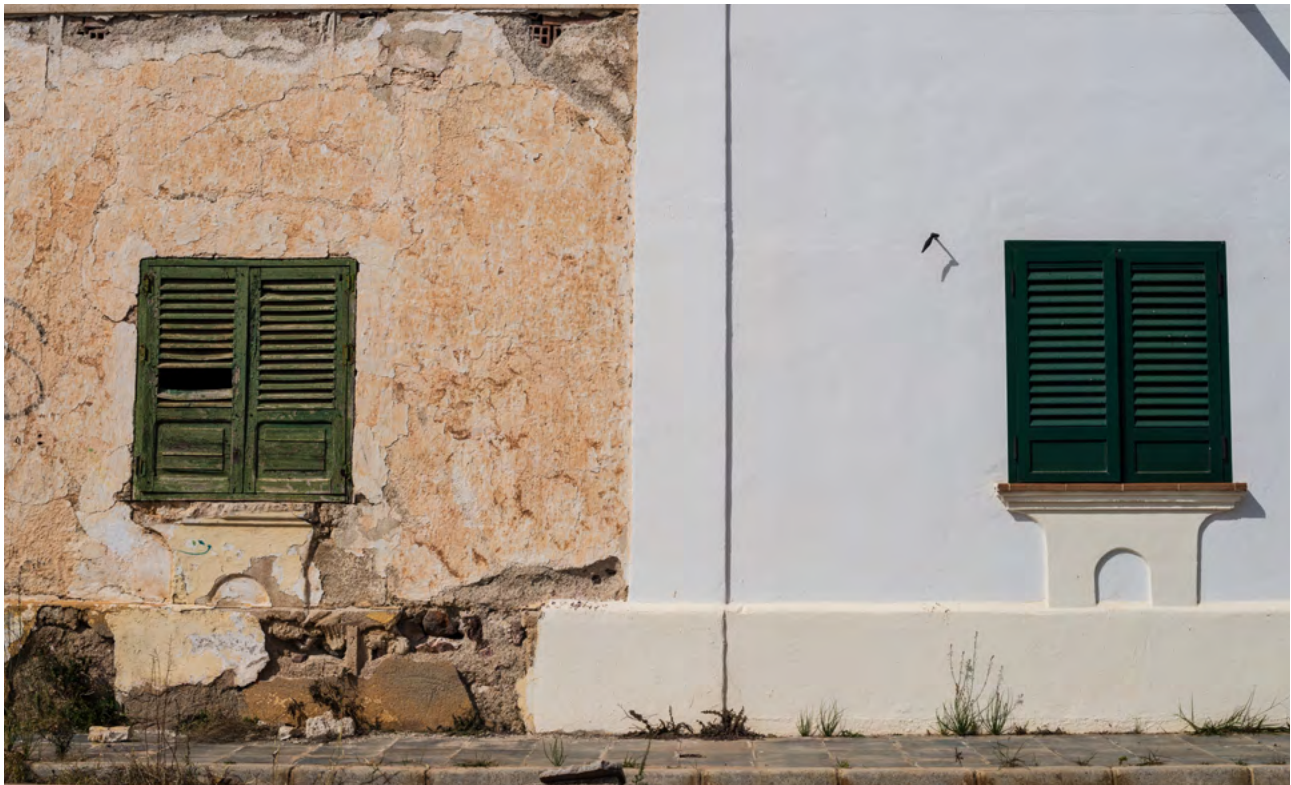
An old vs. new facade
